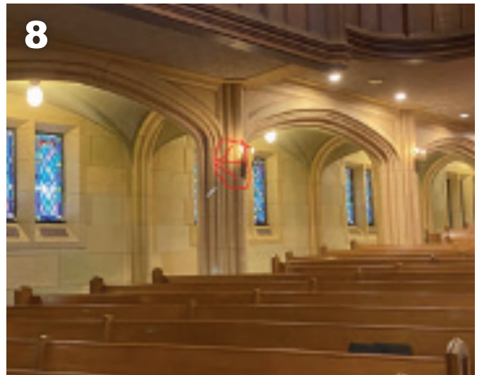
8 Column PTZ Camera location
